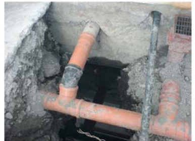
External excavations and vacuum extraction system
