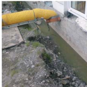
External excavations and vacuum extraction system
